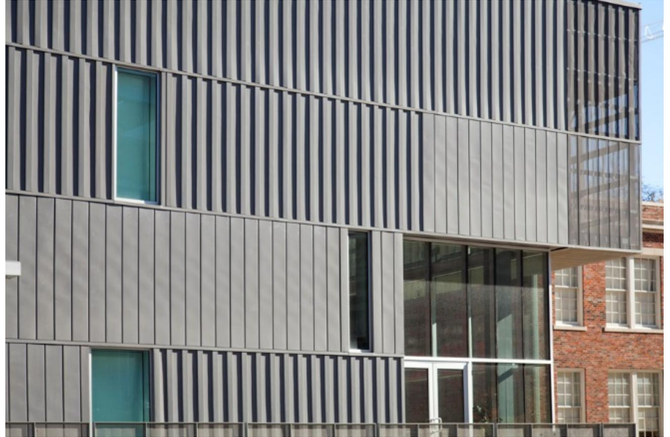
Perforated VMZ Corrugated panel – Metafor panel - QUARTZ-ZINC
