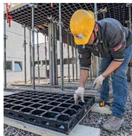
4. Screwing on the new formlining
