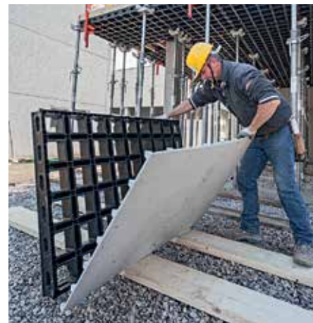
2. Removing the damaged formlining
