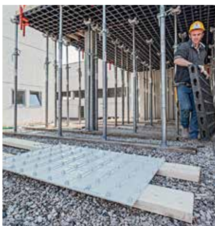
3. Preposition the new formlining
